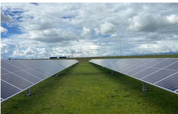
← Solar plant walkways for cleaners and technicians.
